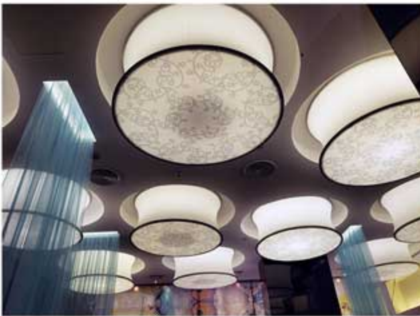
The stretch ceiling lamps are designed exclusively for this project and printed on stretch ceiling by Barrisol® in France.
